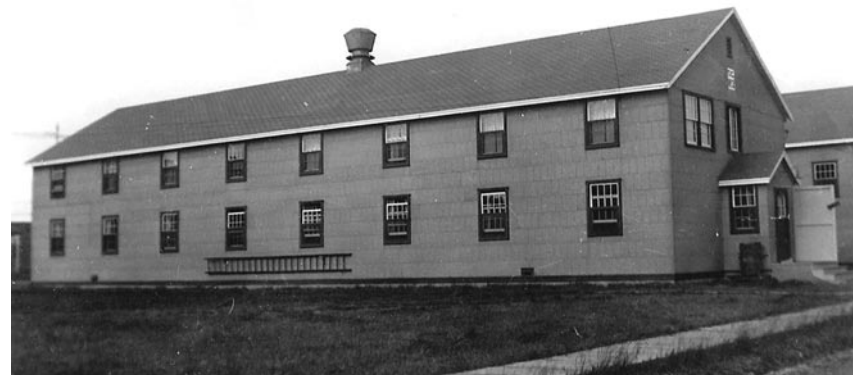
Hazel and the other female radio operators lived on the top floor of the H Building that stood across the road from the hangar.
