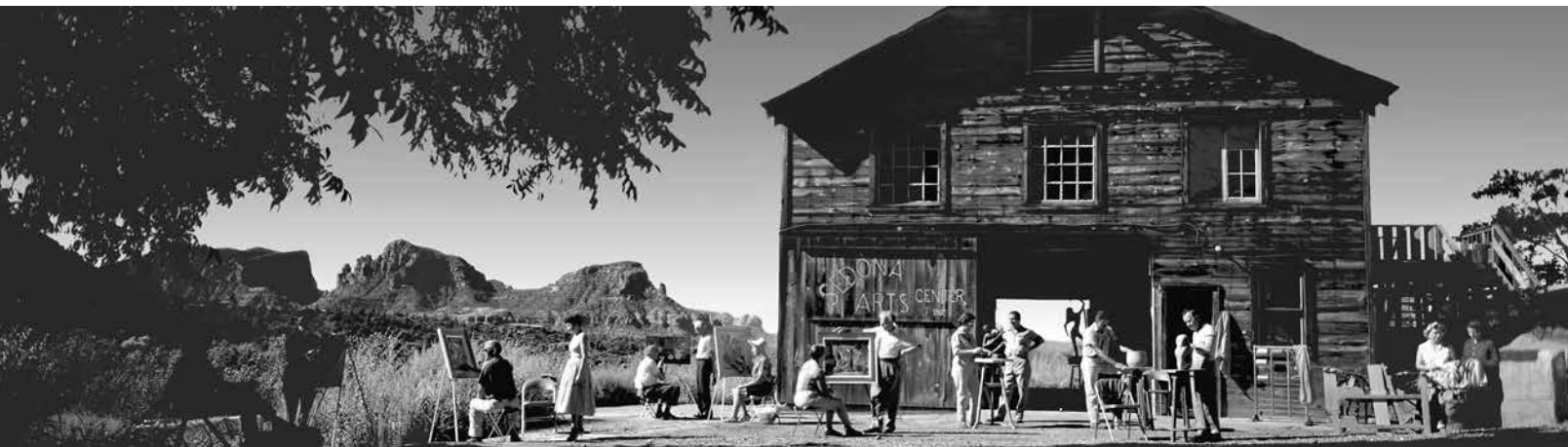
Artists work outside the original Sedona Arts Center in the 1960s. The Art Barn remains the facility's centerpiece.
