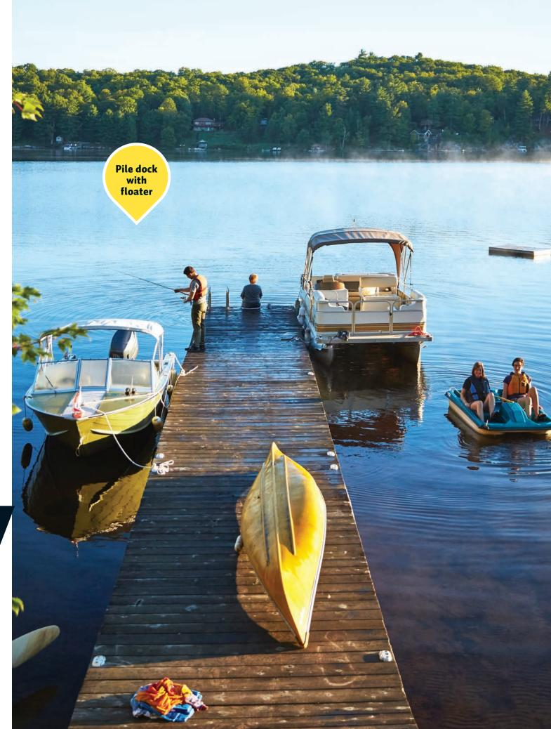
For a mucky shoreline in a shallow bay, Rick Keevil, who has been building cottage docks for more than 50 years, opted for a long dock (on p.77) to allow depth for boats and diving. The first half of the dock is secured with piles drilled as deep as 40 feet into the lake bed. The outer half floats, to save costs and to reduce the impact on lake ecology
